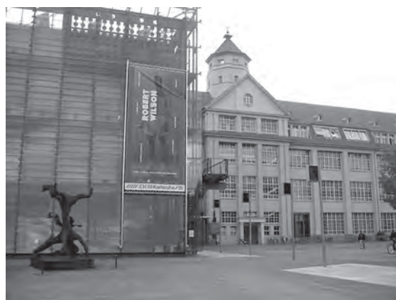
Fig. 1 ZKM Center for Art and Media Karlsruhe
